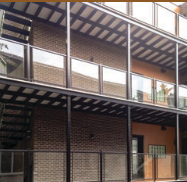
Aluminum Structure Underside
