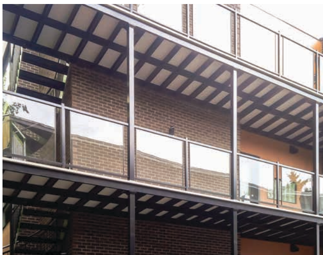
Aluminum Structure Underside
